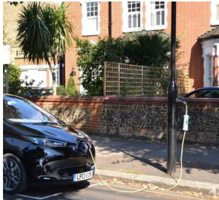
On-street residential charging
